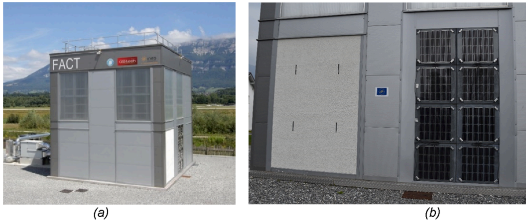
Fig. 4. Photographs of FACT tool (a), of the south-oriented reference wall (on the left side) and of CONIPHER project BIPV wall (on the right side) (b) at CEA site (at Le Bourget du Lac).
