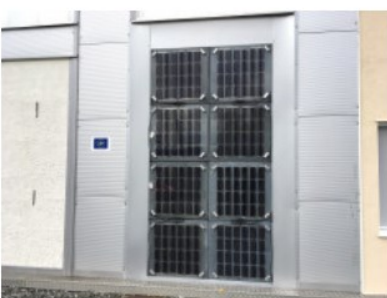
Wiring and finalization of the facade
