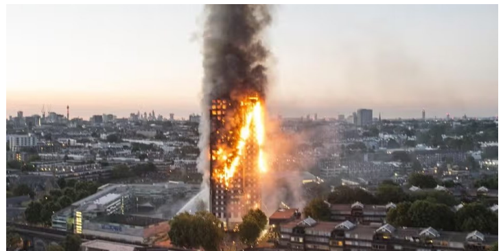
2017 Grenfell tower fire in London
