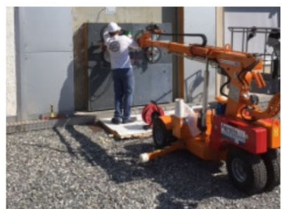
Fixing the panels
