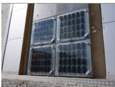
Installation of PV modules
