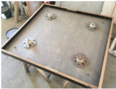
Manufacturing of UHPC facing
