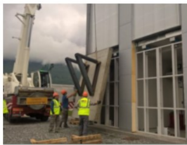
Installation of concrete walls
